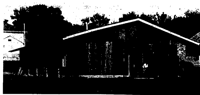
WAYNE MASONS are working evenings to get their new temple ready for the corner stone to be ready for occupancy late this summer or early fall. Laying ceremonies slated for July 6, Nebraska Grand Lodge officers will officiate. The temple, at the corner of Tenth and Lincoln, is expected to be ready for occupancy late this summer or early fall.
